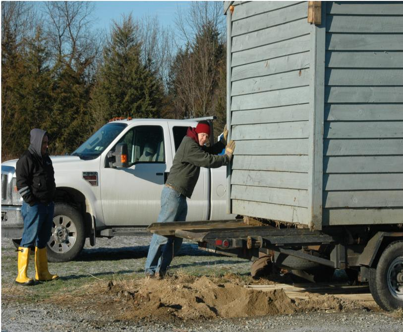
Warren pushing the shed onto the trailer. While this was posed, we really had to do this! The shed was jacked up, and the trailer driven under it, picking it up by the heavy beams that went front to back probably for exactly this purpose. Then the trailer was cranked back up to level, with the shed at the very end. A winch was hooked to the front, and all of us pushed as the winch pulled it forward until it was over the wheels as shown.
