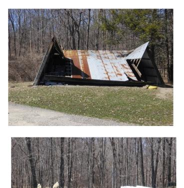
This is the hanger right opposite the ticket booth. The wind pickup up the roof and blew out the walls. It was not too bad but the heavy snow loads this winter brought the roof to the ground. This is on the Top of the list of things needing fixing at the Aerodrome as it houses at least 3 of their vehicles.
